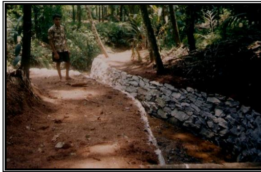
(Photo 3: Nala revetment work undertaken in the project area)
