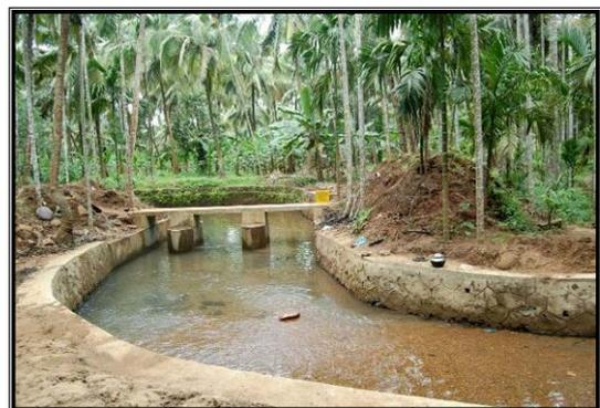
*Photo 1. Canal with stone embankment*
