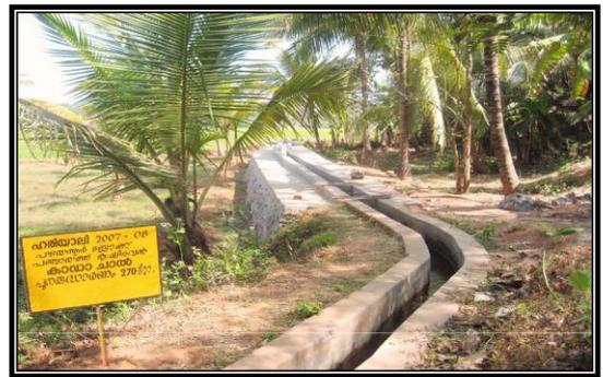
*Photo 2. Canal with stone embankment*
